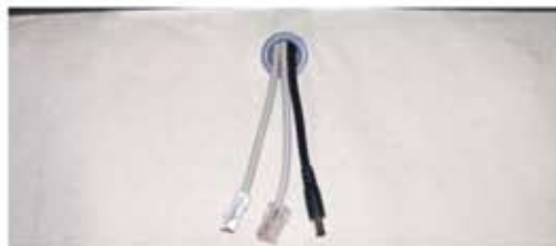
Remote Control and Power Adapter Wires Through Hole Near Head-End (step 5)
